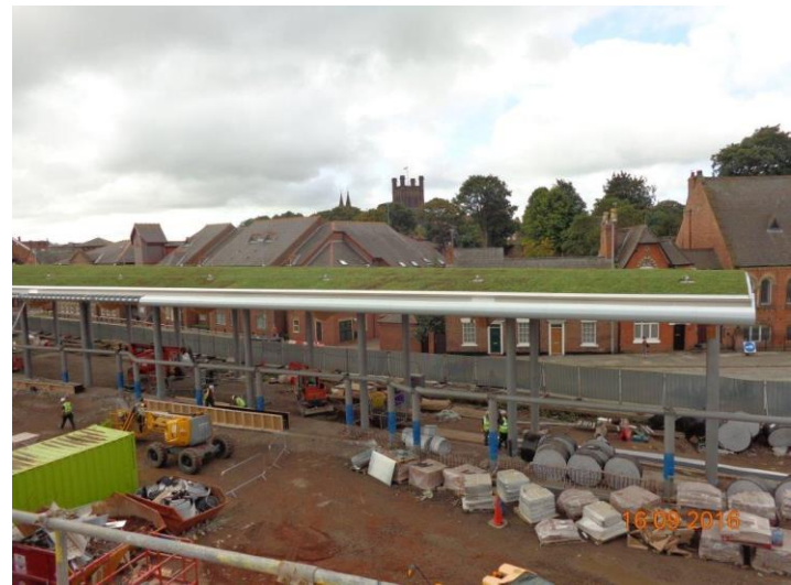
General view of the site
