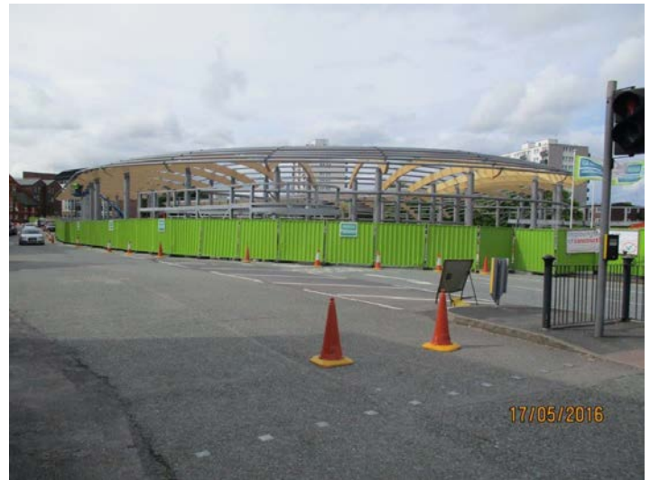
General view of the site (17/05/16)
