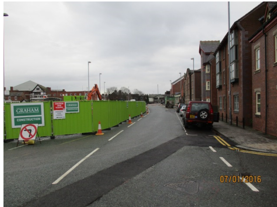
Repositioning of Hoarding to Gorse Stacks
